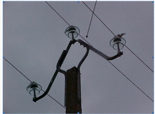
The image shows a close-up of a utility pole armament. A black sleeve is being installed over the metal armament to protect birds. A callout box points to this sleeve with the text 'Armement avifaune gaine'.
